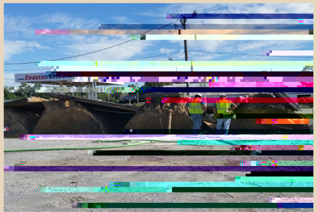
Examples of USTs affected by buoyancy. Hurricane Matthew, 2016. Credit: NCDEQ
